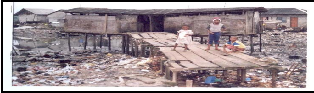
Plate 2: Waterfront Toilet System with poor sanitary and waste management
