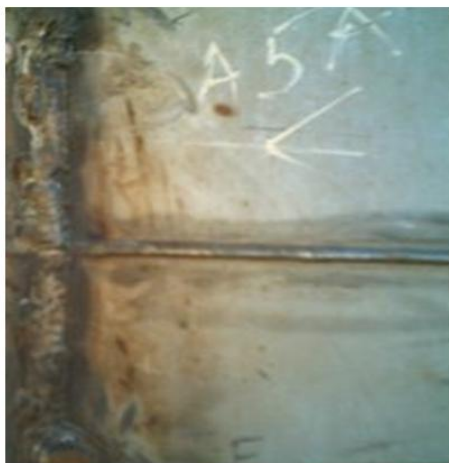
Corrosion on joint due to poor welding procedure
