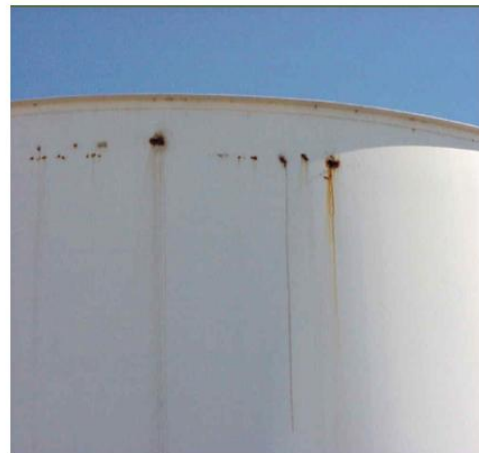
Corrosion starting due to wall failure
